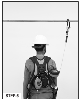
STEP-6 After Lateral Movement Change the SRL's leg for making lateral movement between the anchor points & this can be done with 100% tie-off assurance.
