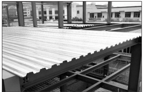
Steel deck and metal roofing
