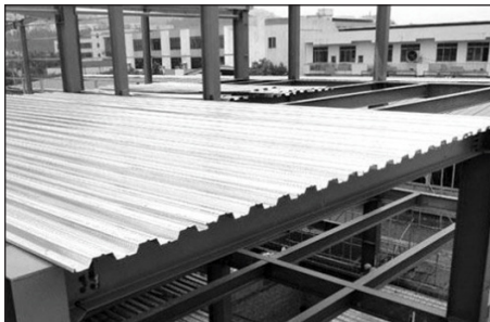
Steel deck and metal roofing
