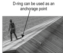
Fig. 3- Now the D-ring can be used as an anchorage point.
