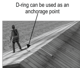
Fig. 3- Now the D-ring can be used as anchorage point.
