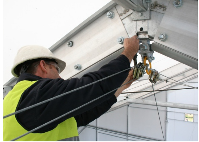
Simple Anchor Points at each end, with no intermediate supports
