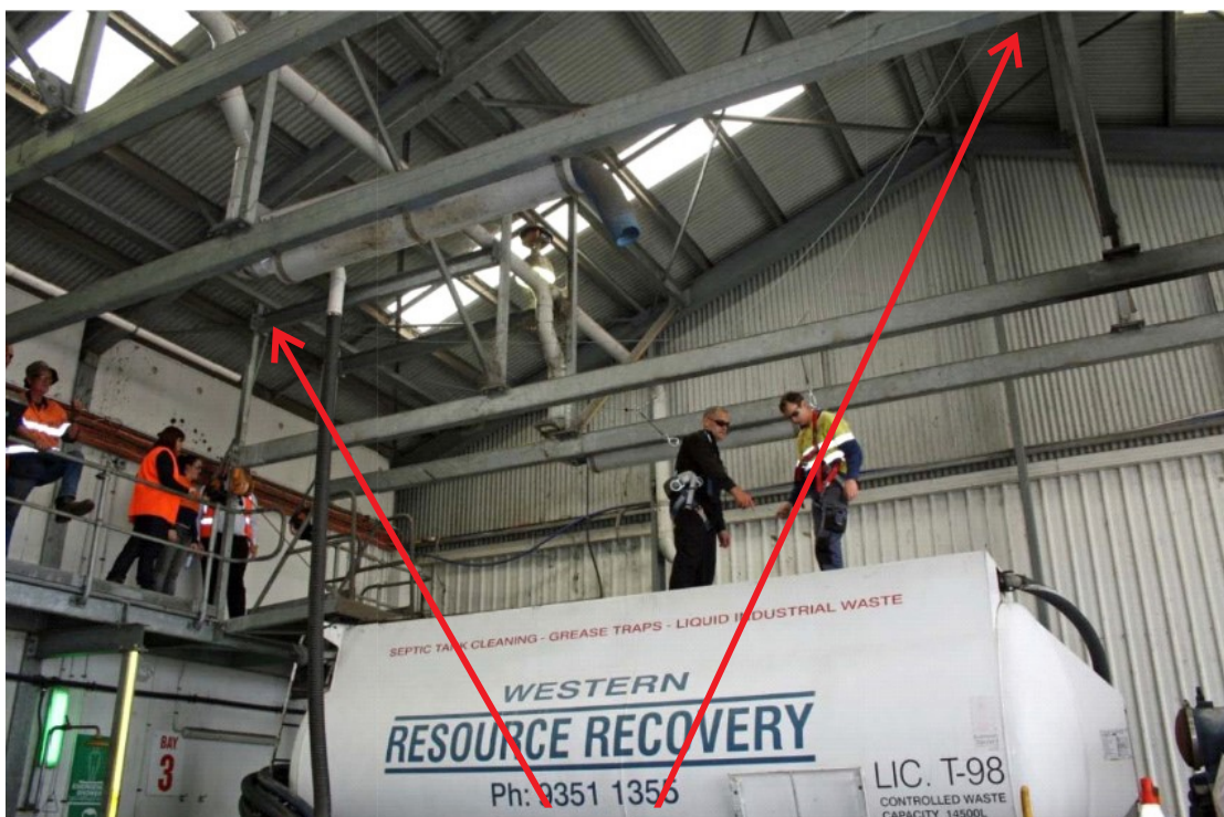
Sloping the roof for installation
