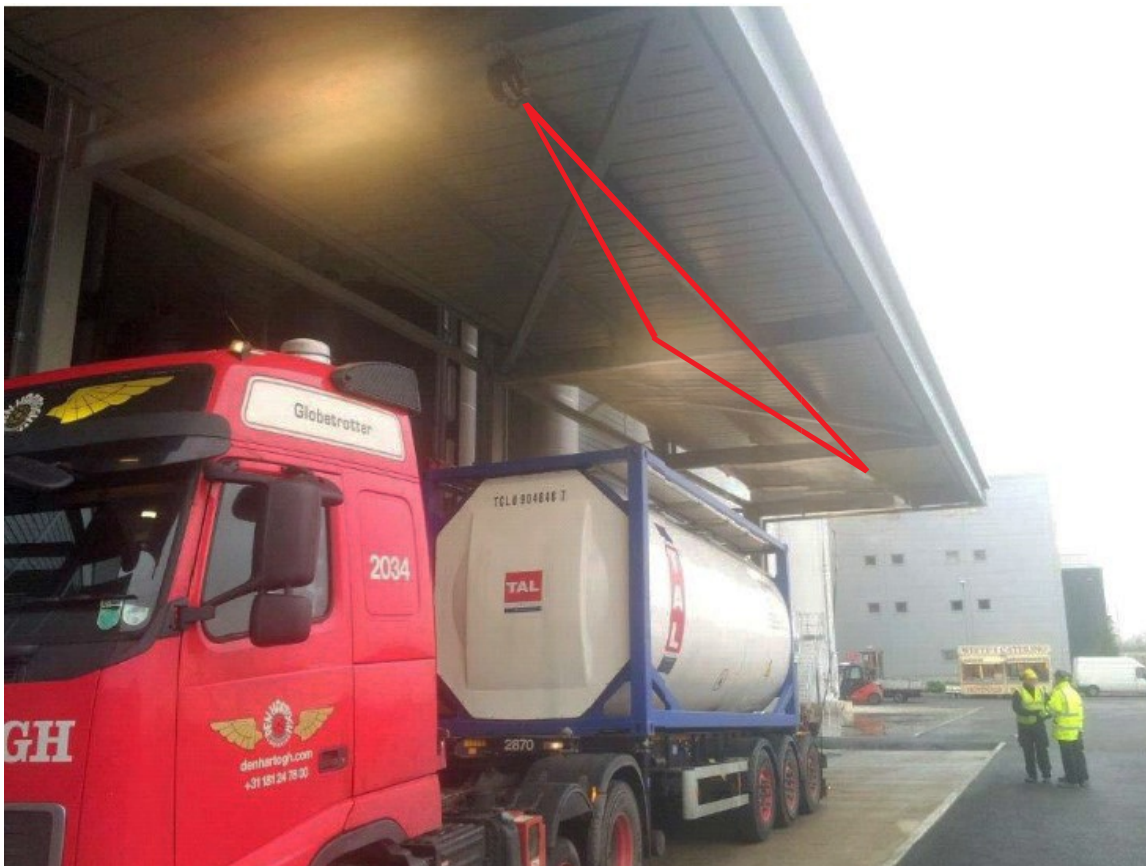
T-Line installed on a 24m long Truck Wash Bay
