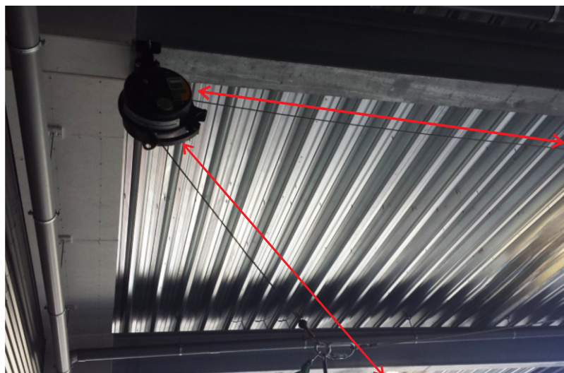
Using the T-Line Beam clamp the installation was straight forward
