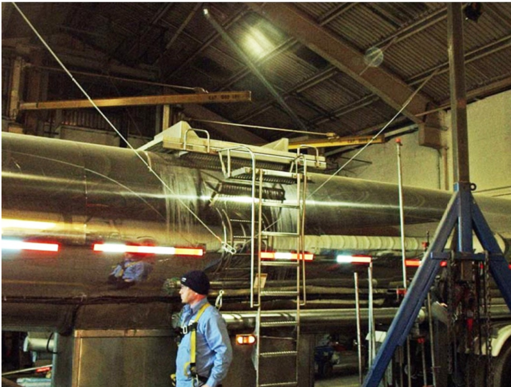
T-Line installed at Tanker Trailer Service Facility – allows the user to hook on before leaving the ground.
