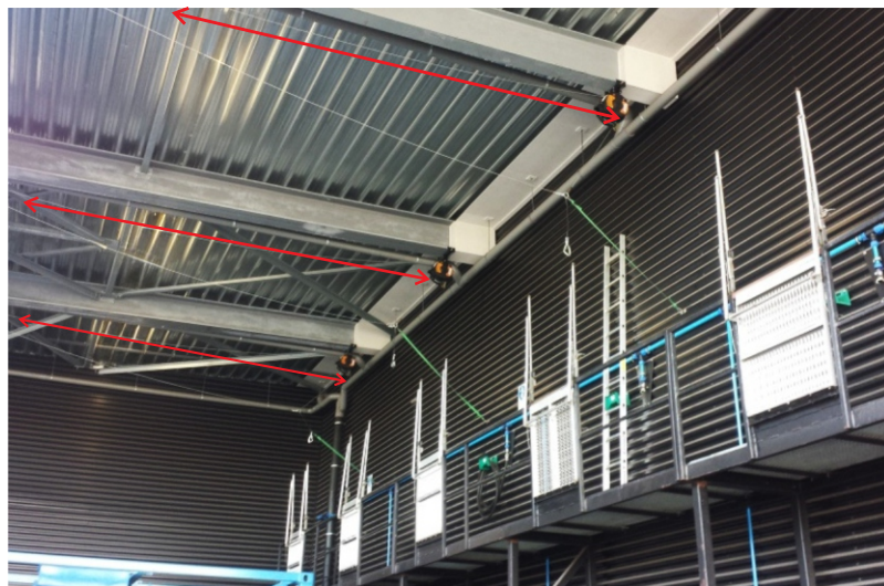
T-Lines installed under the canopy in the 3 bays where access is required.
