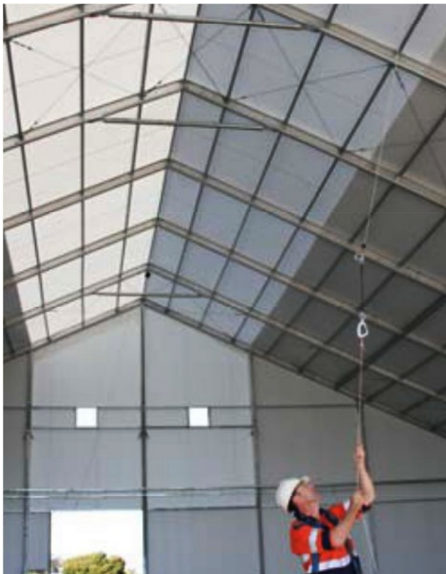
The Lifelines loop around the existing structural braces in the roof, without limiting the movement of the user or the T-Line.
