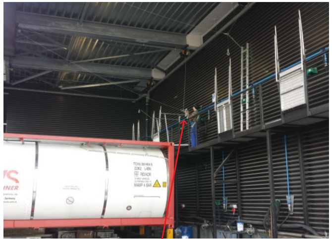
Connecting the T-Line
