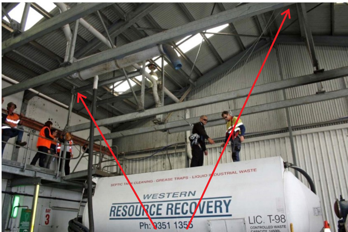
Sloping the roof for installation
