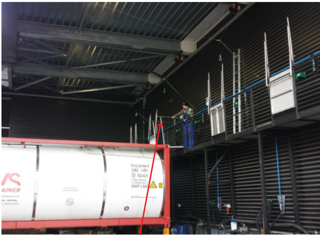
Lowering the Bridge
