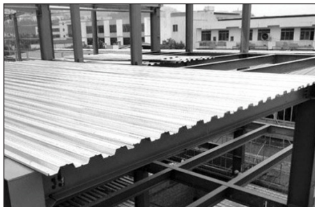
Steel deck and metal roofing
