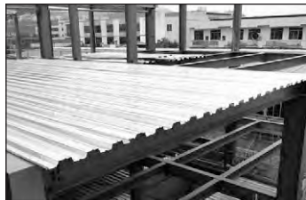
Steel deck and metal roofing
