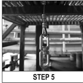
Anchor point below the walkway is ready to use.
