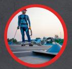
KStrong fixed line systems are made of corrosion-resistant stainless steel. Some components are also CED-coated for greater protection. Our systems are thus warrantied so long as the system is inspected annually and maintained after inspections by a KStrong Certified inspector according to requirements of EN 365.2004.
