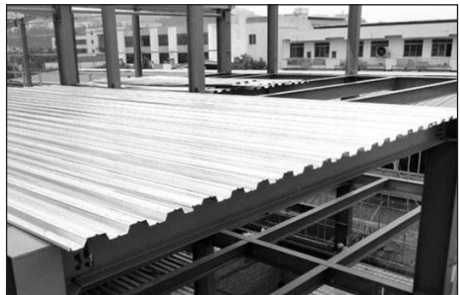
Steel deck and metal roofing
