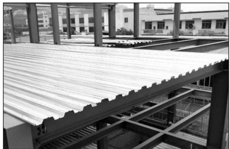
Steel deck and metal roofing
