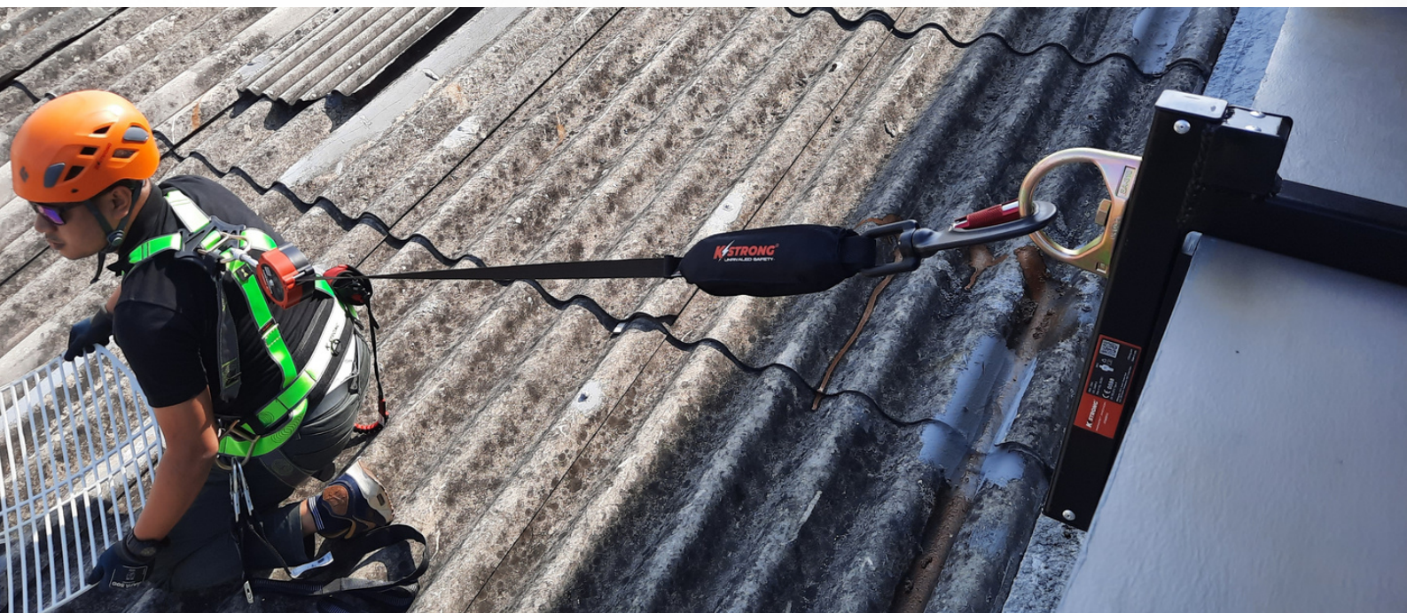
REMOVABLE CONCRETE ANCHOR C/W SLEEVE 15KN (AFA930310)
