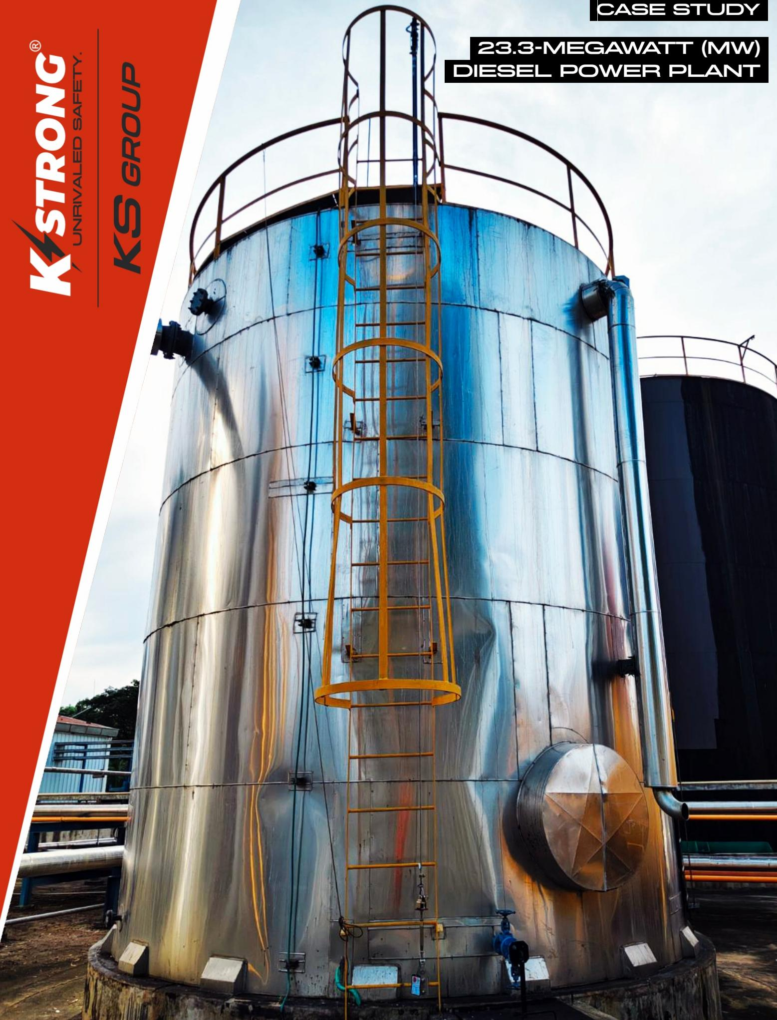
VERTICAL LIFELINE SYSTEM FOR DIESEL TANK FARM
